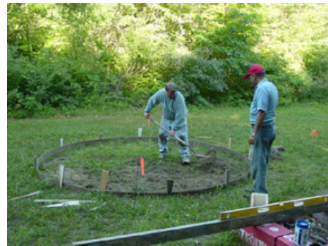
preparing the platform
